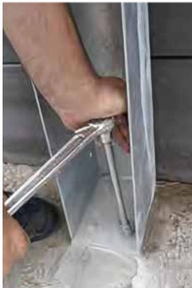
The gap between the panels and the columns is normal. When the pool is filled with water, the panels will touch the columns due to the force of the water.
