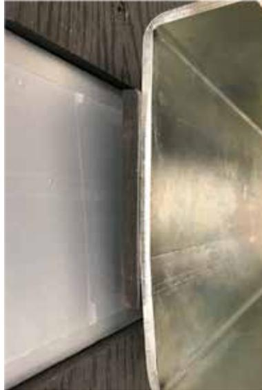
Place the pillar along the junction rail. Drill the screed vertically with a drill equipped with a 10 mm Ø concrete drill bit, using the pillar as a template.
