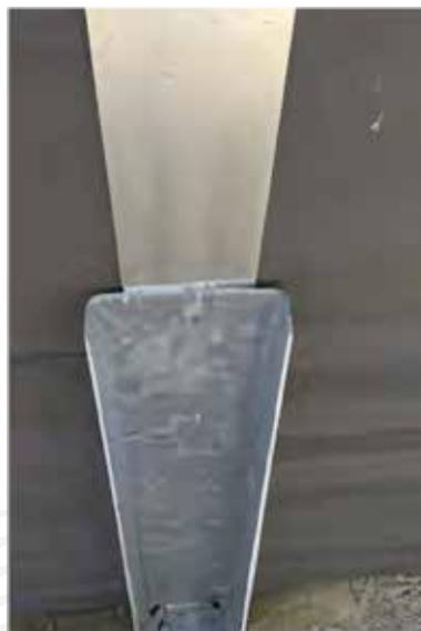
Insert the composite board supplied in the kit between the junction rail and the metal pillar.
