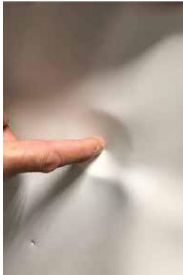
At this spot, cut a circle in the center that is smaller than the hole for the discharge nozzle. To make this cut in the liner, you can also make a cross with a cutter and then cut the outline.
