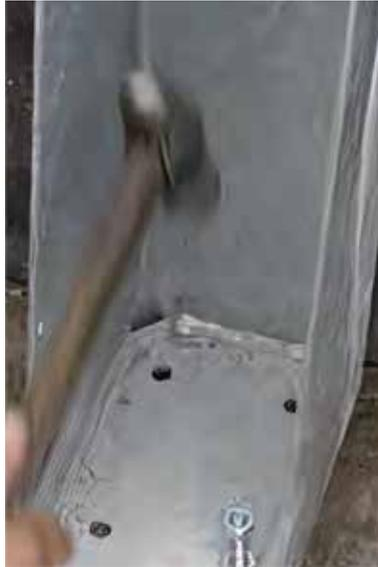
Tighten the 4 nuts firmly in a cross pattern.
